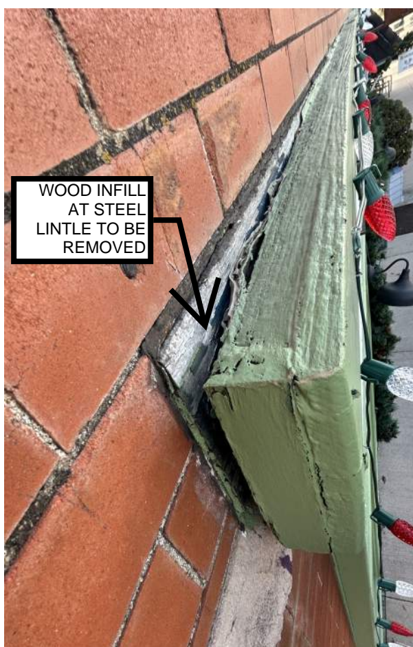
FRONT FACADE STEEL LINTLE PHOTOS NOT TO SCALE
